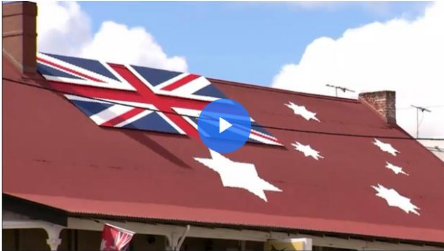
Pub facing demolition over Australia flag
