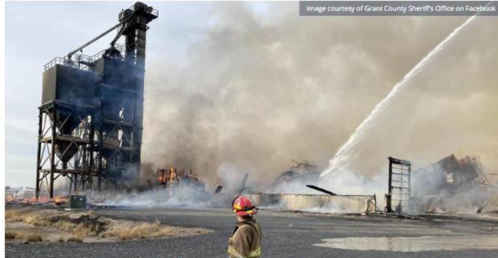
A view of the collapsed walls of the Wilbur-Ellis fertilizer plant near Moses Lake, WA.
