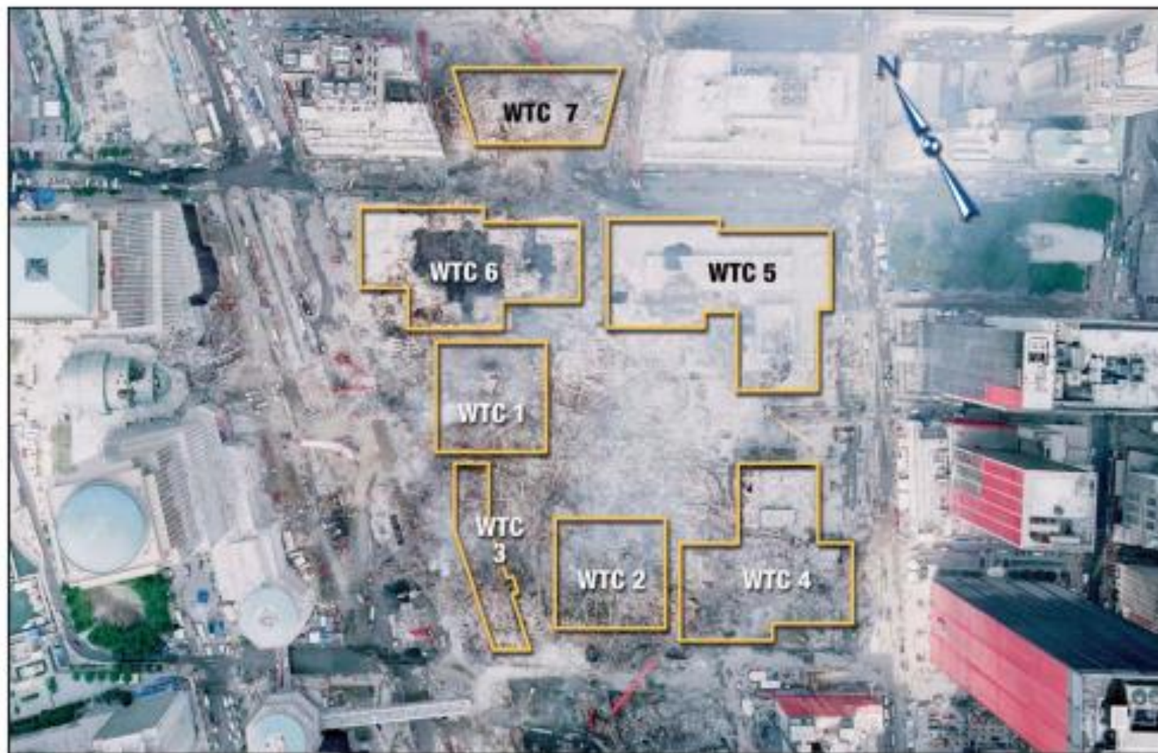
Figure 2-23 Aerial photograph of the WTC site after September 11 attack showing adjacent buildings damaged by debris from the collapse of WTC 1.
