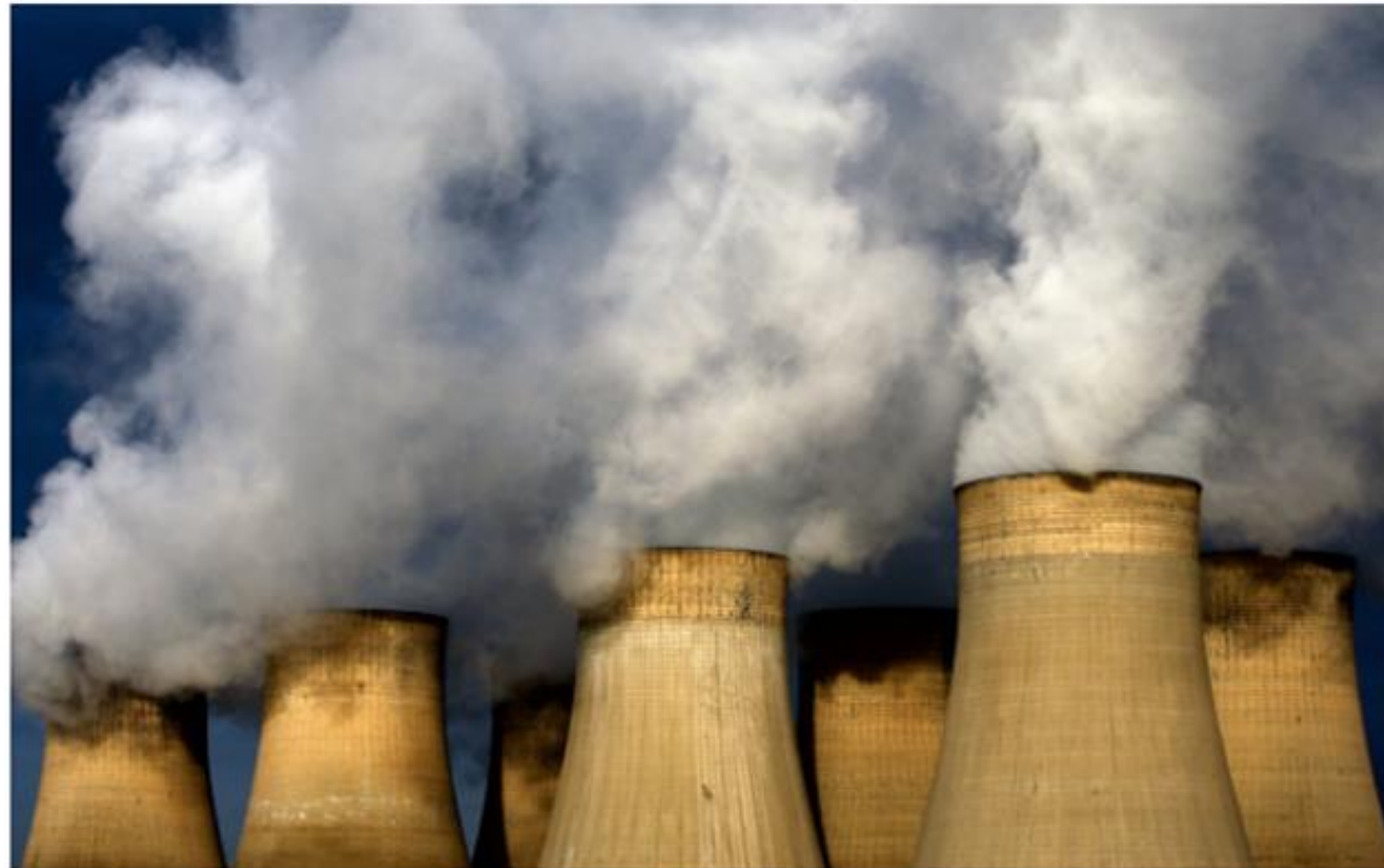
Uniper's Ratcliffe-on-Soar coal power plant in Nottinghamshire started producing electricity for the first time in weeks on Monday morning | CREDIT: David Davies/PA
