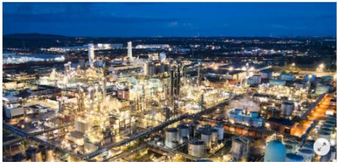
Chemical park OQ Chemicals in Oberhausen
