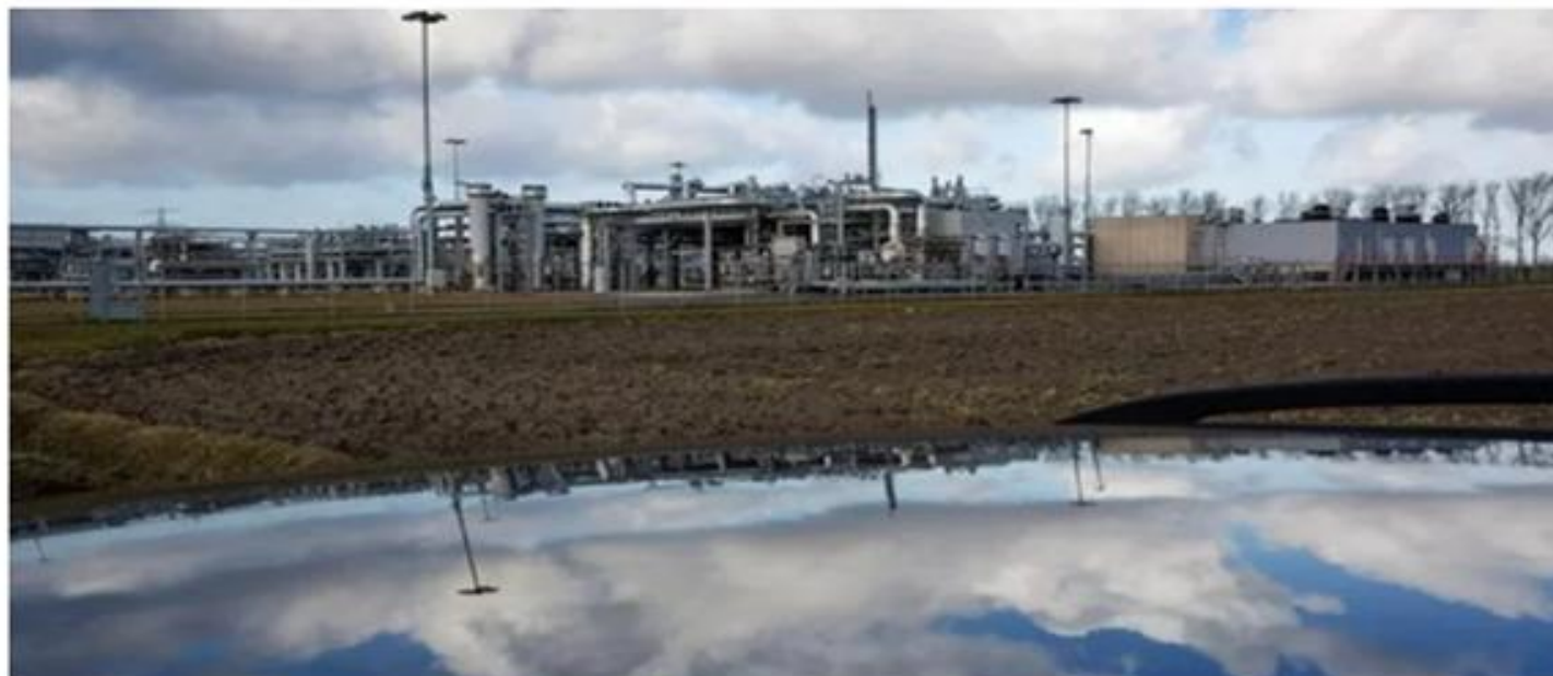
Gas infrastructure at Groningen gas field (Photo: reuters.com)
